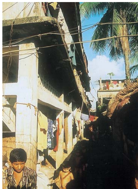
Slum in three storied building, Sylhet
